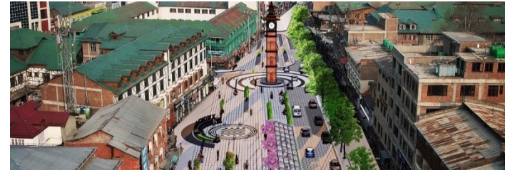
According to the smart city officials in Srinagar, the five-year project plan started in 2018 for which funds of around Rs 1000 Cr were allocated for various
